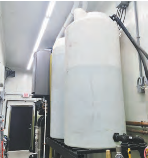
Two large water tanks are included in the utility room between the two bays. One holds water directly from the Panora water system. The other holds water that has been channeled through both water softener and reverse osmosis equipment to produce "spot free" rinses.
