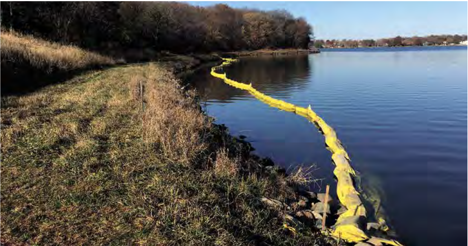
Work began near the ski team dock and will move west. The crew is doing 1,000-foot sections of shoreline at a time. A debris curtain about 300 feet long in the water is being used to contain any loose grass or debris that may fall into the lake as the shoreline rip rap is repaired.
