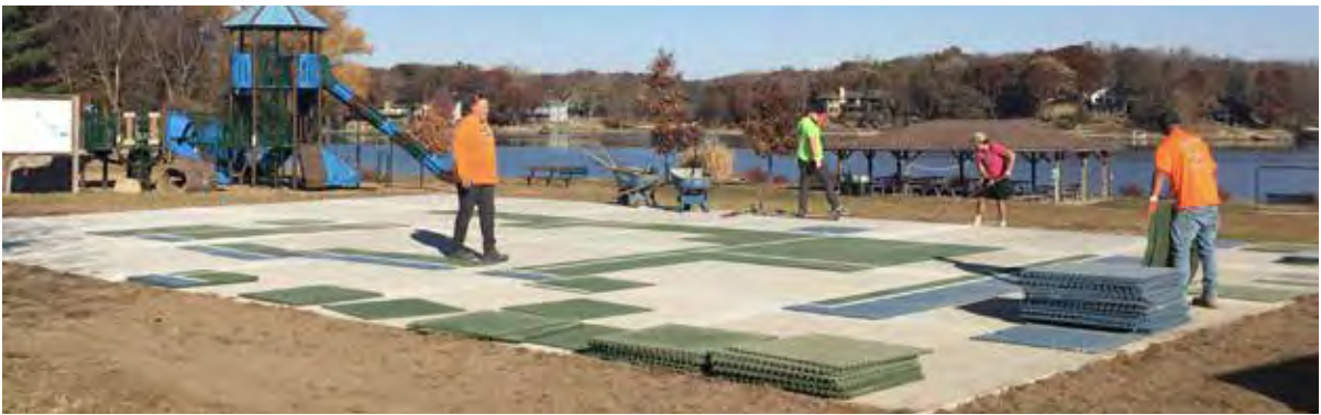
The new sports court at Sunset Beach will accommodate both basketball and pickleball. On Oct. 31, Bryan Jansen of Sports Construction Midwest and his crew placed sports tile on the 40-foot by 60-foot concrete slab and installed the anchor for the basketball hoop system. A fence around the court will be finalized in November, then a portable pickleball net added. South Shore trail enhancements and the Friends general fund. A coupon to complete and send with a donation is available in an ad on page 16. Donations by check can be mailed to Friends at P.O. Box 488, Panora, Iowa, 50216. Direct donations can be sent via Venmo @Panorama-Friends. Donations also can be made by credit card online at www.friendsoflakepanorama.org . Details about other ways to donate, plus all past, present and future Friends projects also are on the Friends website. ■
