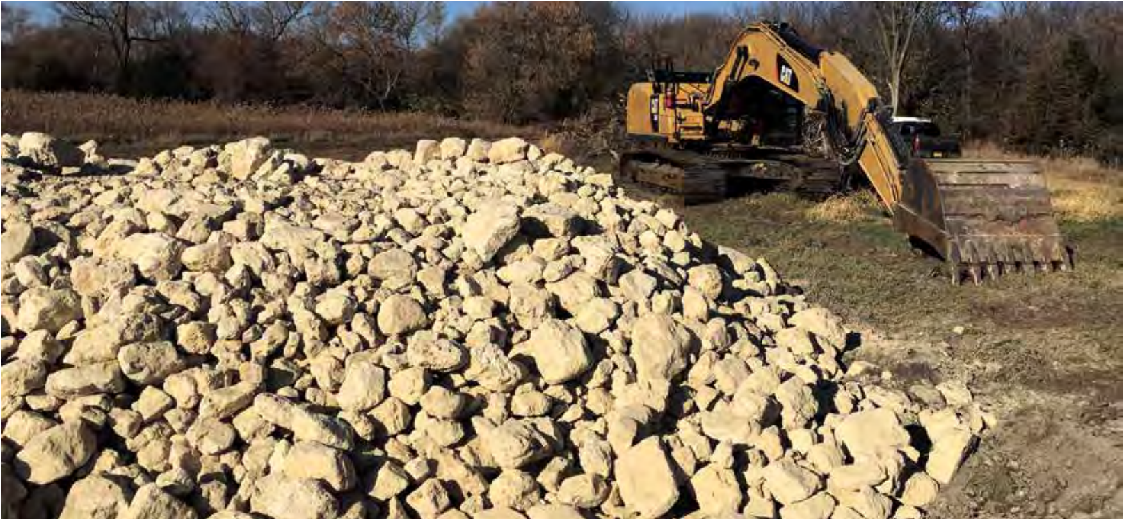
Dolomite rocks are shown piled on Lake Panorama's south shore as a project to repair rip rap along the shoreline began the end of October. JNC Construction of Clearfield is doing the work, which is expected to last six to seven weeks.
