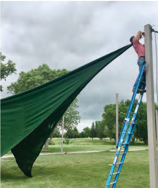
Installation of the two fabric sails took about two hours. On July 7, the sails were attached to the six poles that had been installed earlier in concrete footings.
