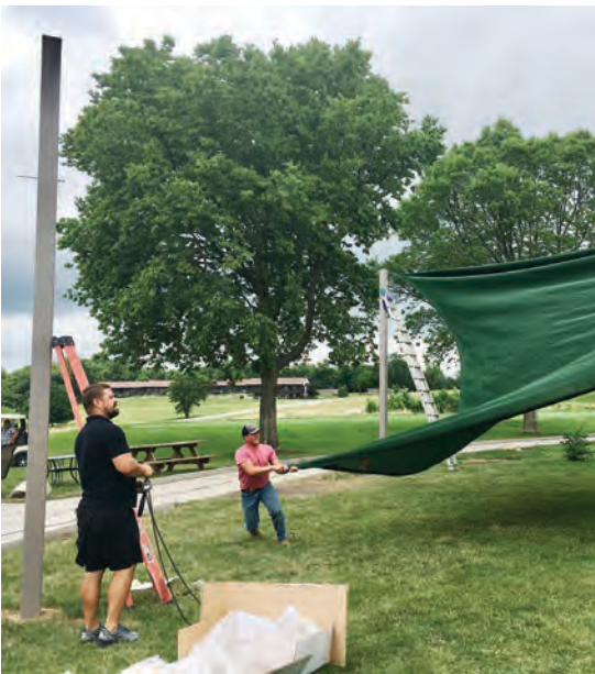
Sam Pieczynski, owner of Shade Sails of Iowa, watches as the first sail that had been attached to two poles is stretched to reach a third.
