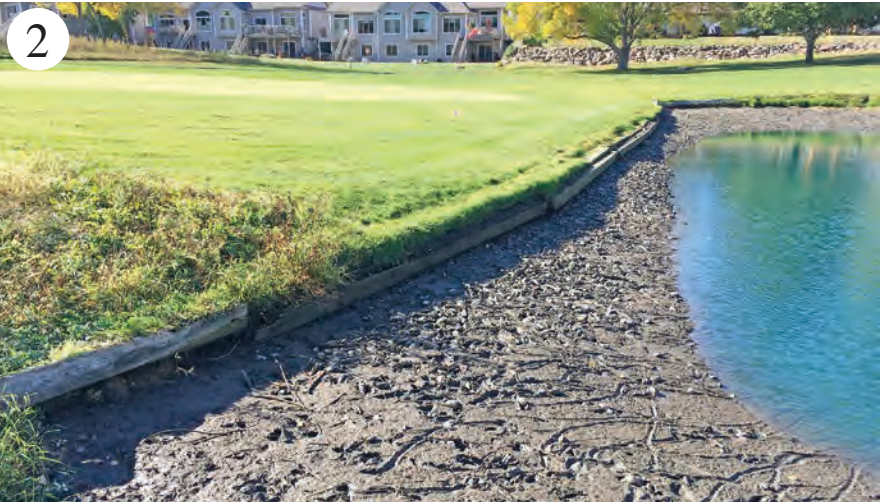
An old wall made of railroad ties had been deteriorating for several years.
