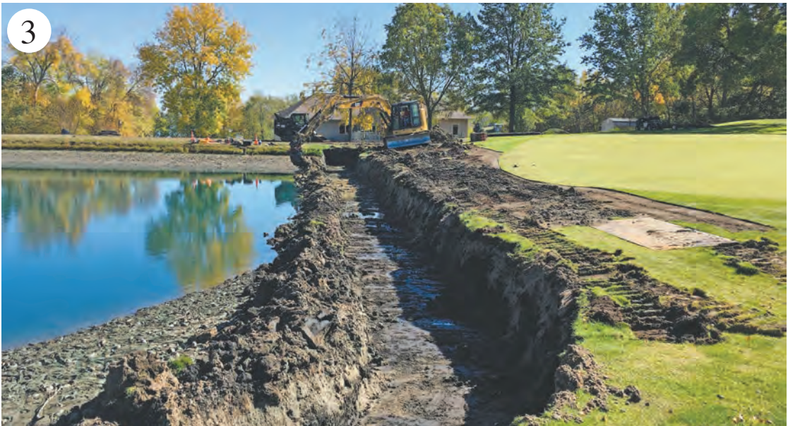
Once the old railroad ties were removed, a wide trench was created.
