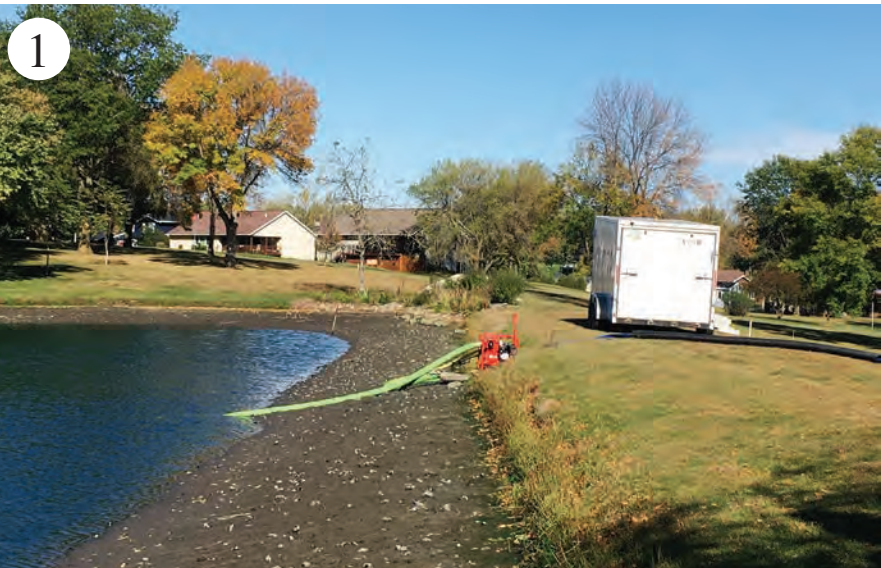
A pump was used to partially drain water from the pond before construction could begin.
