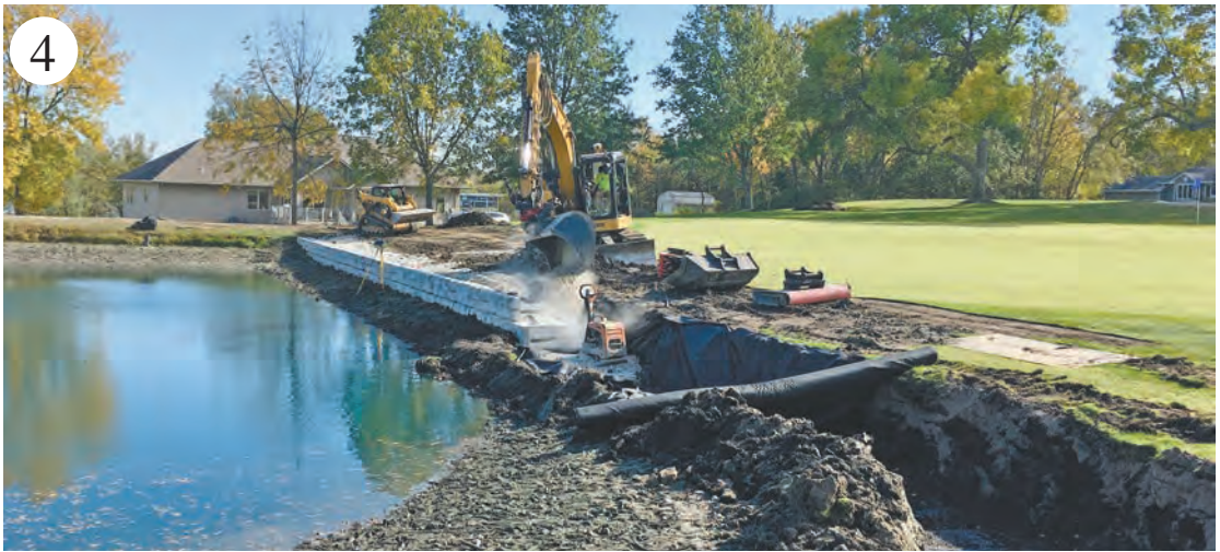
A retaining wall was built using pre-cast modular concrete blocks that “lock” together. The area between the block wall and the green was backfilled with dirt and gravel.
