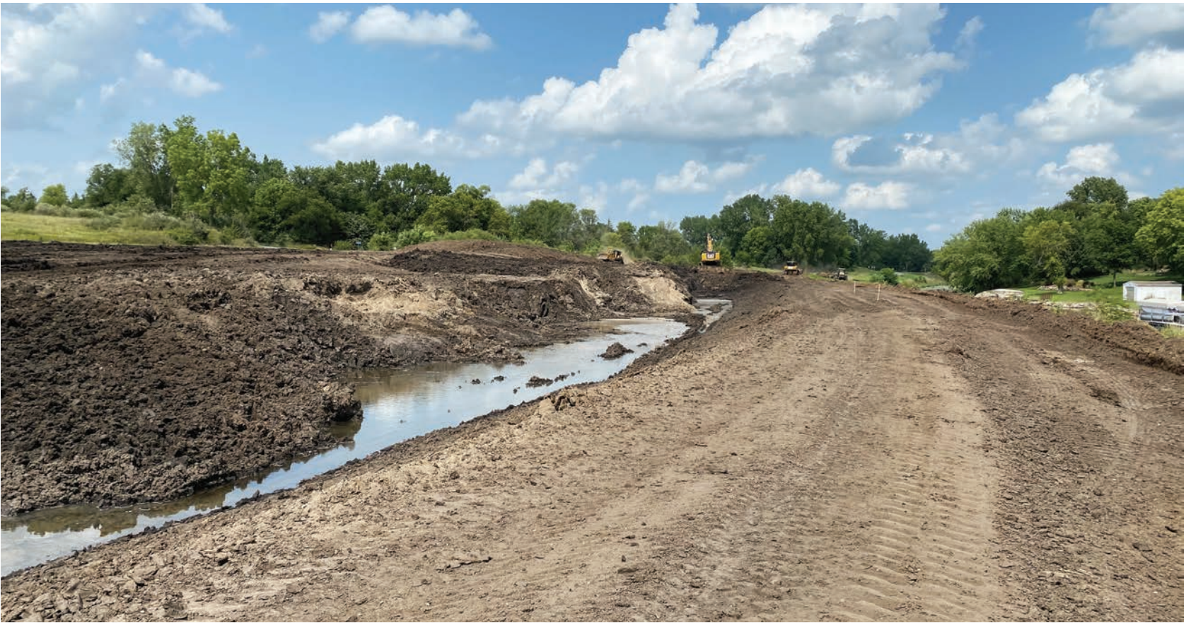
This “bench” created along the west shoreline of the stream that enters Burchfield Cove will be used by LPA crews as they dig sediment from the stream with a long-reach excavator.
