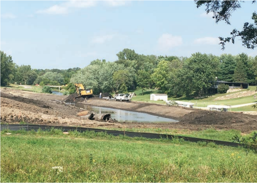
The Burchfield stream project, financed by the Lake Panorama RIZ, involves the construction of a bench on the west side of the stream, with an adjacent pit to accommodate silt removed from the stream. Once the dirt work is complete, 1,700 feet of the west shoreline will be rip rapped with limestone.
