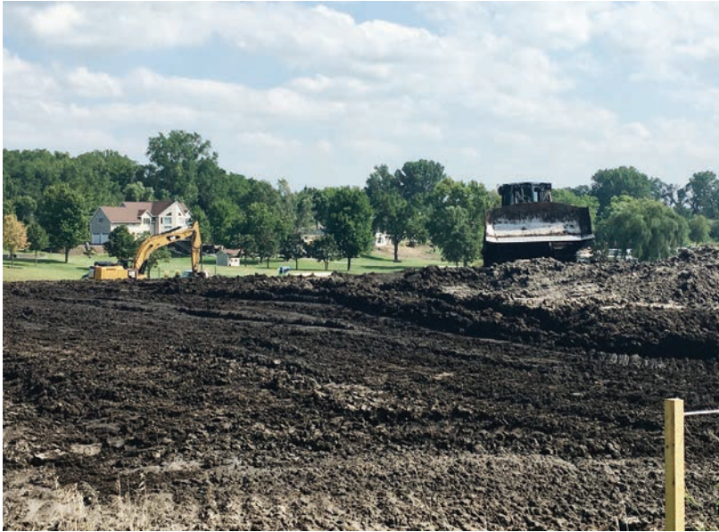
Many tons of dirt have been relocated recently during a project near the mouth of Burchfield Cove. An old silt basin is being rebuilt between the stream and Panorama Drive to better accommodate sediment dug from the stream.
