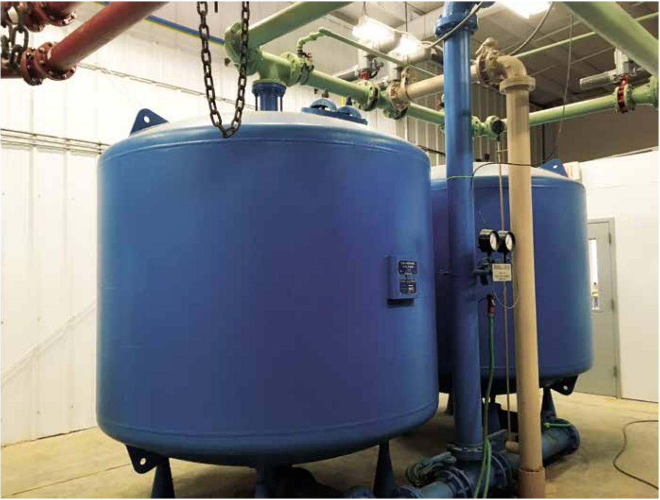
One part of the existing water plant building was filled with these large blue gravity water filters. During December, contractors removed these along with other old pieces of equipment and pipe. This area now is being used for some components of the new system.
