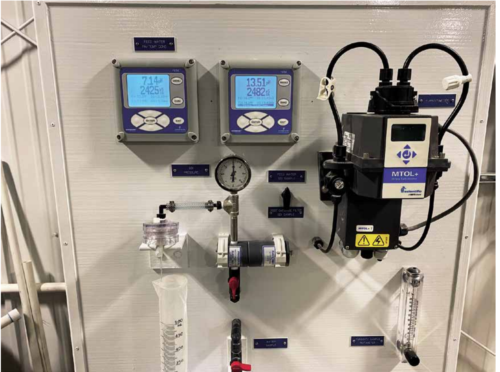
A control panel for the RO system is along the back wall of the addition built to accommodate the new system. It provides constant information on the operating status and includes several taps so water can be drawn and tested as needed.
