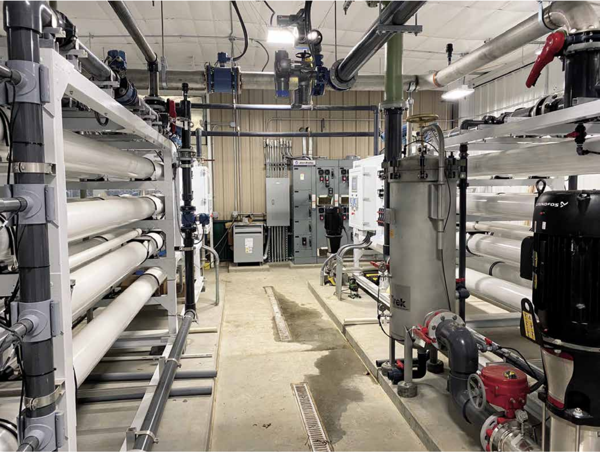
The reverse osmosis (RO) system involves two sets of 12 white tubes. These tubes are the heart of the reverse osmosis process. Water runs through the tubes twice, using eight the first time and four the second. Once that process is complete, 20 percent raw water is mixed in to come up with the finished product.
