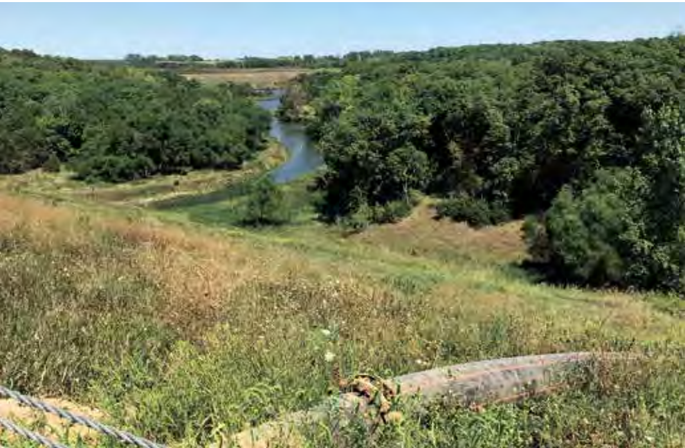
All summer, a large pipe has snaked from Lake Panorama's upper basin up the hill and under the road to the county basin, carrying silt and water pumped from both the LPA dredge and the Dredge America dredge.
