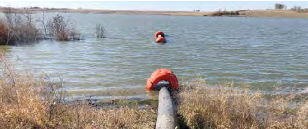
This photo was taken in early November from the same spot as the April photo. It's easy to see how the water level in the silt basin rose over the summer with so much silt and accompanying water being pumped from two dredges.
