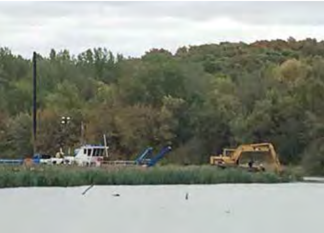
Heavy equipment removed vegetation from a large island south of the Fansler Bridge. This then allowed the Dredge America's cutter head to take over, digging out the island down to the river bottom.
