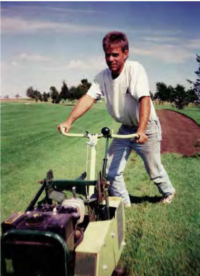
The golf course was built without cart paths. For several years, Wollner used an 18-inch sod cutter, making four passes per hole, to create 6-foot-wide cart paths. The paths then were covered with gravel.
