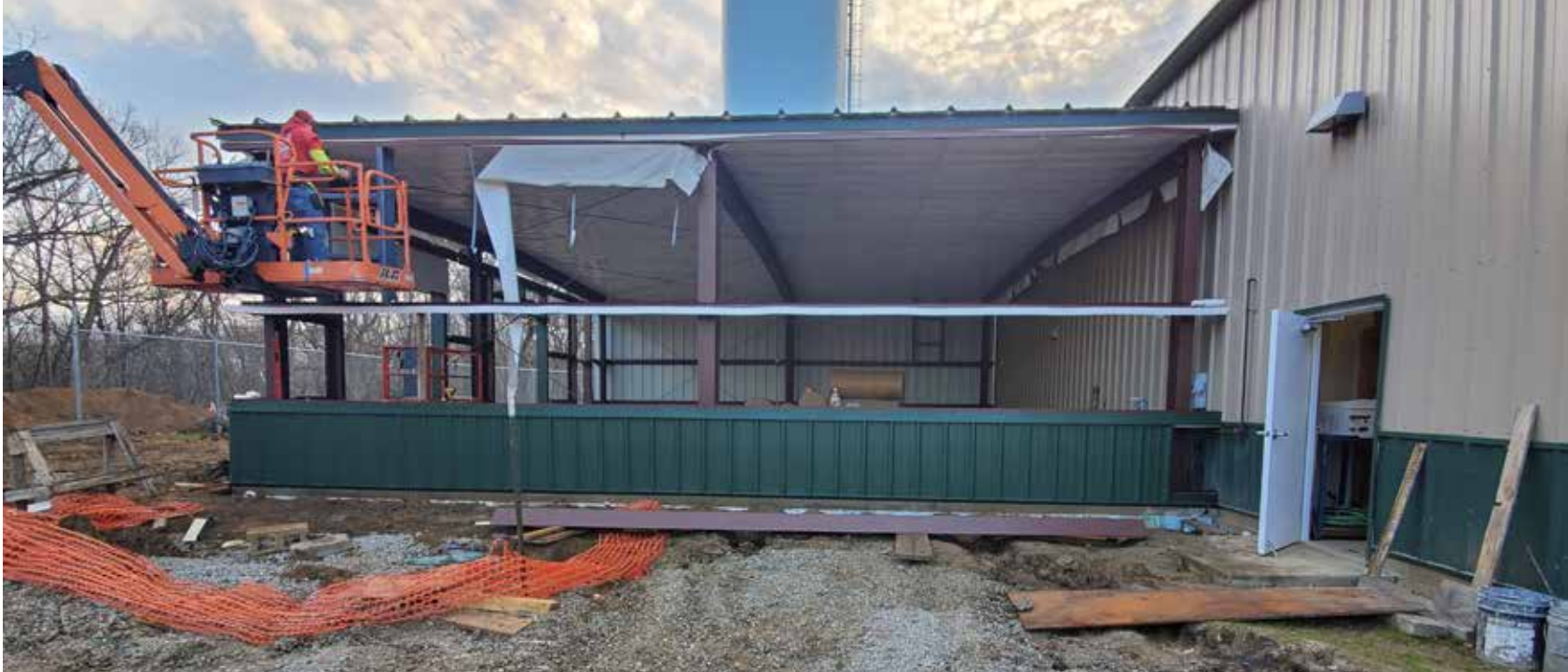
A 40-foot by 40-foot addition to the existing water plant building was constructed to house the reverse osmosis equipment.
