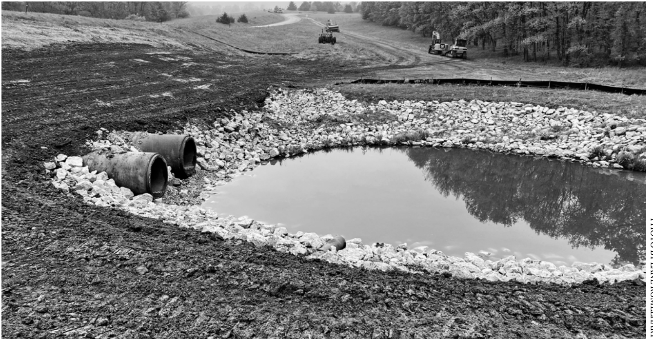
Once the tubes were reconnected, a drainage tile was built into the dam bank to pull seepage out of the bank and direct it to the lake. The final step was regrading the surface of the silt dam and restoring it with grass seed.
