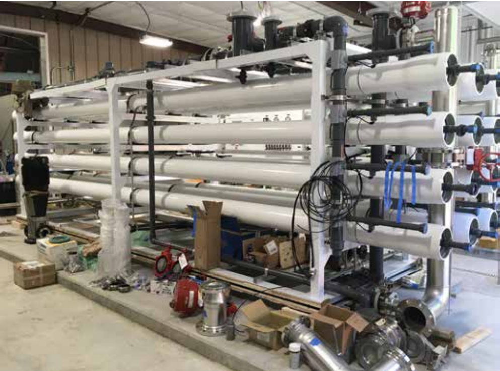
These white tubes are the heart of the reverse osmosis process. Water runs through the tubes twice, using eight the first time and four the second. Once that process is complete, 20 percent raw water will be mixed in to come up with the finished product.
