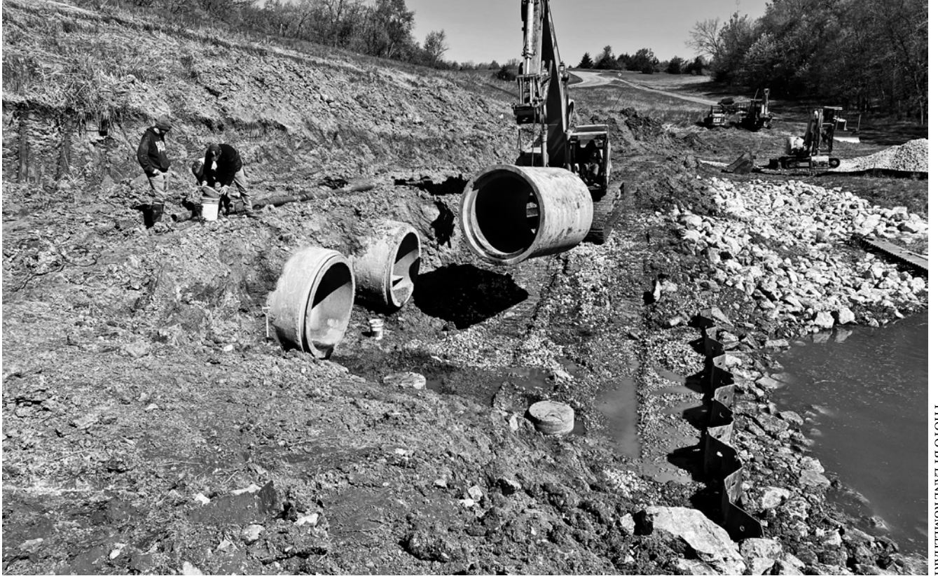
Some repair work at the west end of Jones Cove was completed earlier this year. The concrete tubes running under the road had begun to pull apart and needed a stronger foundation. This was done by driving sheetpile straight down at the edge of the cove. Limestone rock was added behind the sheetpile for backfill. Next the surface was graded and the concrete tubes put back in place.
