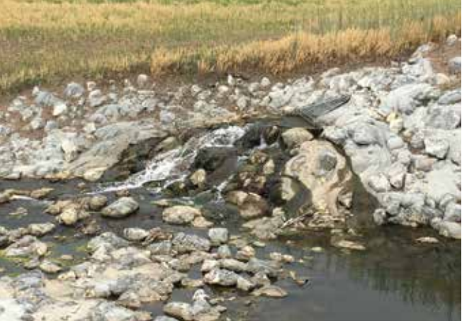
Water comes through the wetland outlet structure and spills out onto a rock bed on its way to the creek that leads to Burchfield Cove.
