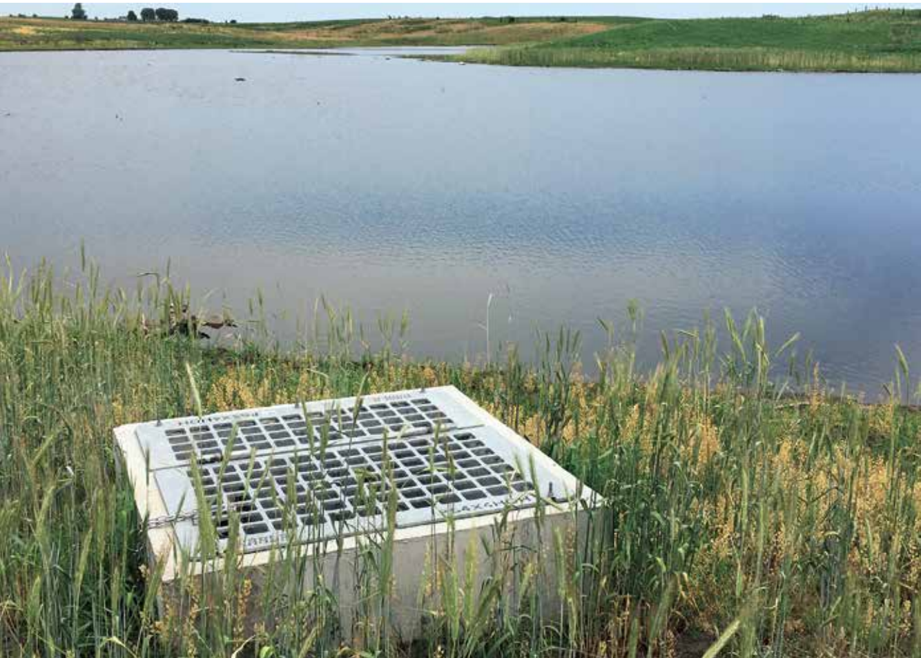
This square concrete box with a metal grate is an inverted pipe that houses the wetland control structure. It contains a channel with stop blocks that are added or removed to taper the water level of the wetland. Flow levels are adjusted seasonally.
