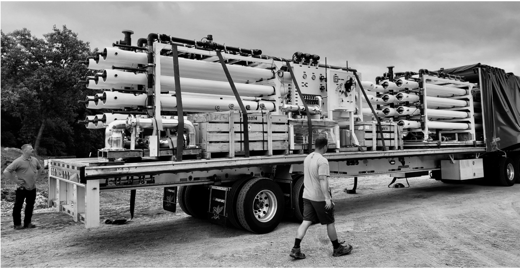
The two large components of the reverse osmosis system arrived by truck and had to be lifted by a crane into the new building addition at the water plant.
