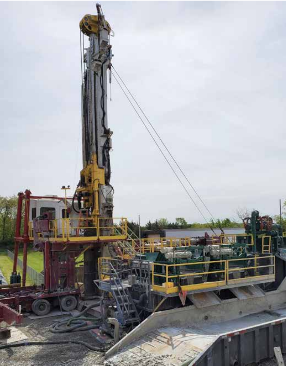
Drilling a second Jordan well on the grounds near the LPA water plant was done in late May. When the water plant upgrades are complete, only Jordan well water will be used, and two Dakota aquifer wells will be closed.
