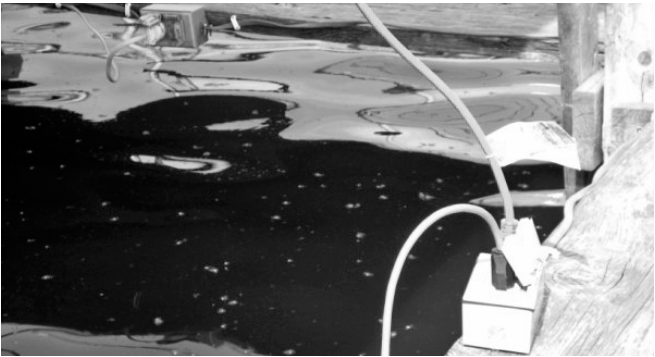
These photos provided by the office of the Iowa State Fire Marshal/Electrical Bureau are examples of unsafe uses of electrical wiring, outlets and cords on a boat dock.
