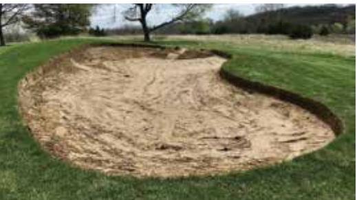
This photo shows the bunker near the eighth green at Panorama West after all existing sand and gravel was removed, and the perimeter outlined with a straight cut. This was before new drainage was installed, followed by new gravel, a 2-inch layer of capillary concrete, and new sand.
