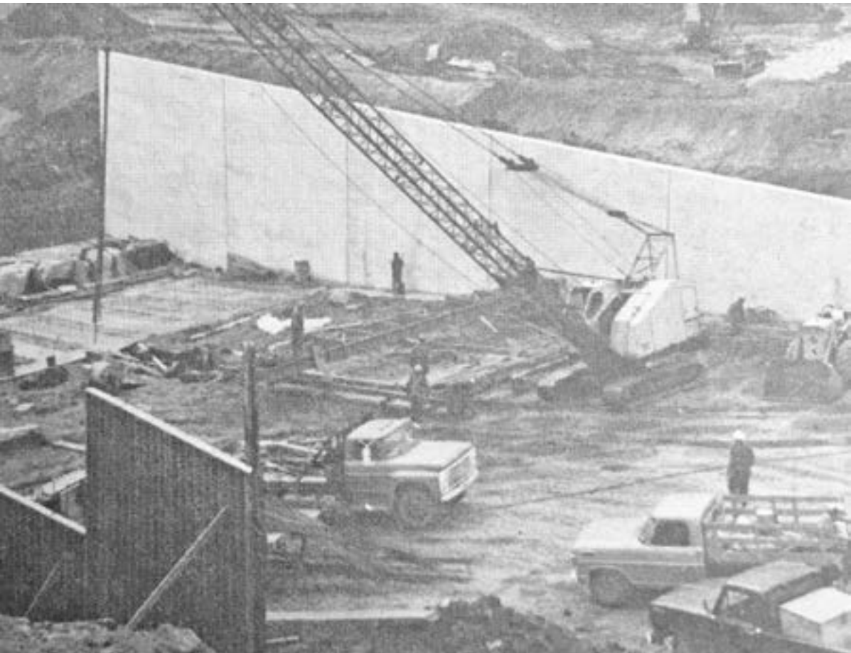
Construction on the dam got underway in 1969. Here workers are preparing the grade in the floor of the spillway chute prior to installing forms and reinforcing steel.
