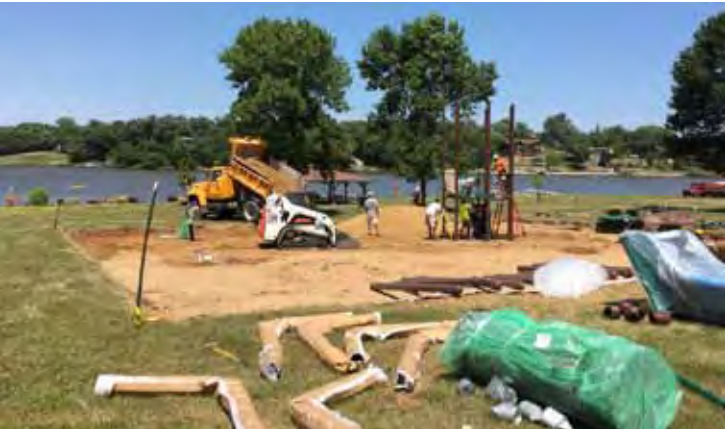
The main tower was the first to be built as playground construction got underway July 11. LPA staff assisted the project by preparing the site, and delivering and spreading pea gravel to form the base.
