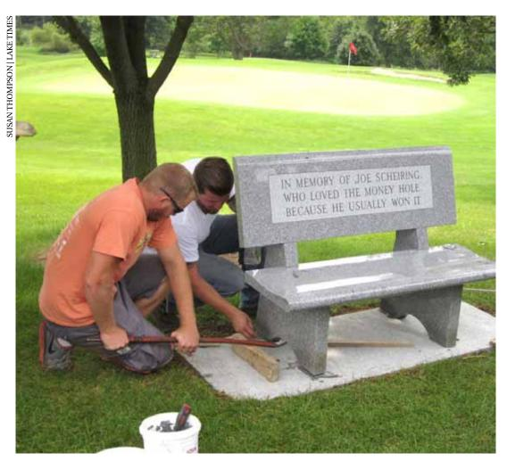
Two new granite benches were installed August 5 at the Panorama West golf course. The work was done by Des Moines Winterset Monument. Each bench was placed on a granite pad with a sand base underneath, then secured to the pad with a special epoxy.
